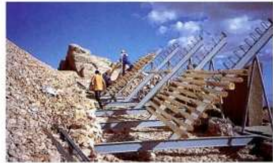
Fig. 2. The snow barrage under construction (photo: A. van As).
