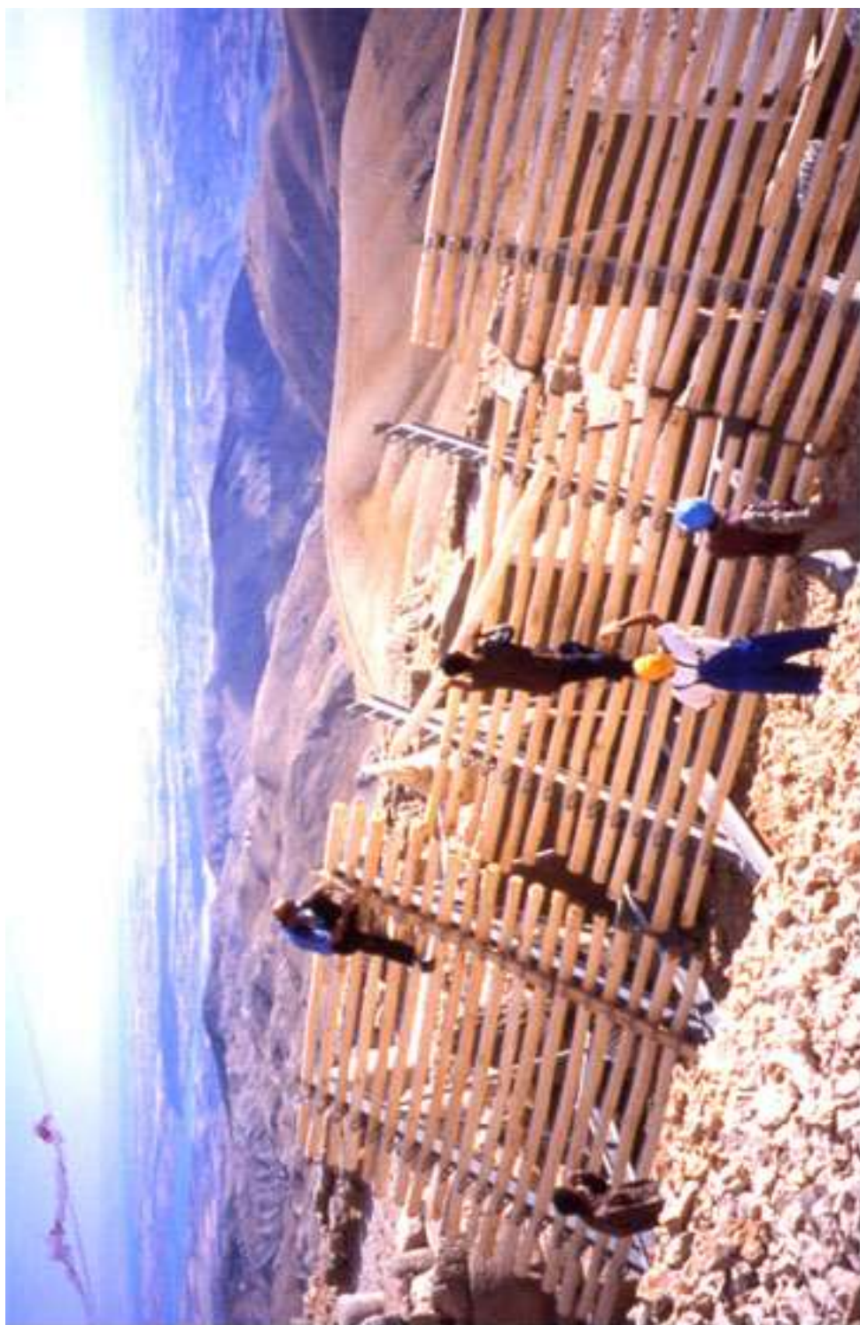
Fig. 16. The snow barrage at the back of the row of sandstone stelae in the north-eastern section of the West Terrace. It was constructed in July/August 2002 in order to prevent the three standing stelae from falling down during the next winter.
