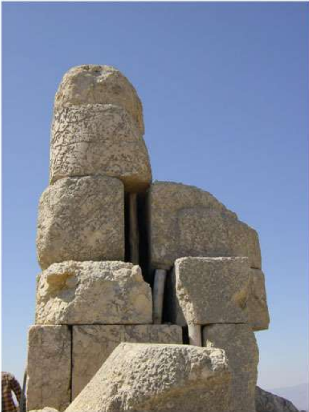
Fig. 11a. South side of the statue of Antiochos (C) on the East Terrace, showing the awkward position of the blocks, temporarily supported by wooden poles. Situation in August 2002.
