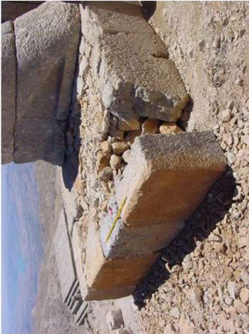
Fig. 13b. Northern plinth of guardian eagle and lion (H-I) on East Terrace, seen from northwest. Limestone blocks, forming the four sides of the plinth, placed in their original position; part of one block (L. 138) is missing. Filled up with local limestone pieces and grout (see above). The five blocks belonging to the three lower courses of the eagle statue (H) are replaced in their original position. Situation in August 2003.
